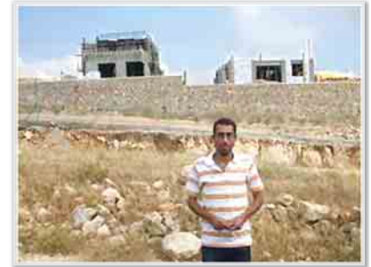
◆ Bassel Araj lives with his parents and siblings in a house 100 metres from the pictured construction site in the illegal settlement of Gilo. (Photo credit: ©Joe O'Brien/EAPPI)
